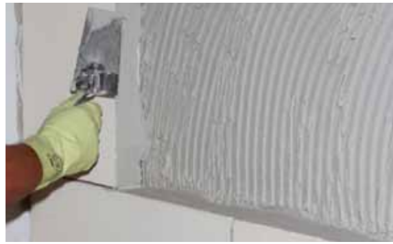
A bead of KÖSTER Hydrosilicate Adhesive SK is applied along edges of the boards to make sure that the joints are fully filled.
