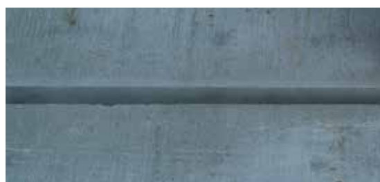
Cleaned joint flanks
