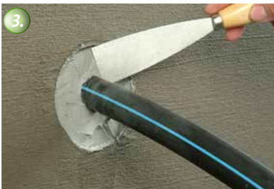
To protect the waterproofing the area is smoothed and protected with KÖSTER KB-Fix 5.
