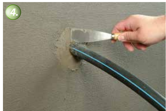
The pipe penetration is now permanently waterproofed.
