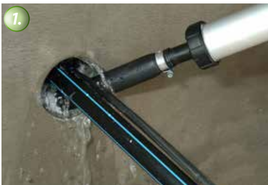
KÖSTER KB-Flex 200 can even be used under flowing and pressurized water.
